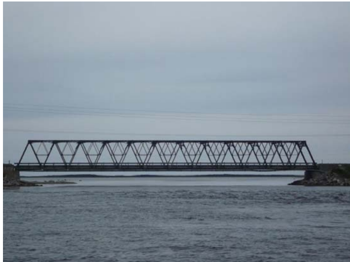
Route 430 bridge over St. Paul's Inlet
